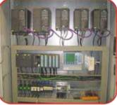
VFD Panels are designed to control the speed and torque of electric motors by varying input frequency and voltage to motors. VFD Panels are used as energy cost savings are especially pronounced in variable torque centrifugal fan and pump applications where there is larger power reduction for a relatively small reduction in speed.
